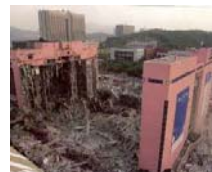
•Department Store Collapse
